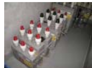
Capacitors containing PCB
