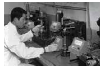
Electronic Micrometer—1961 Anritsu developed its checkweighers from the technology it created with this early micrometer that measured object dimensions.
