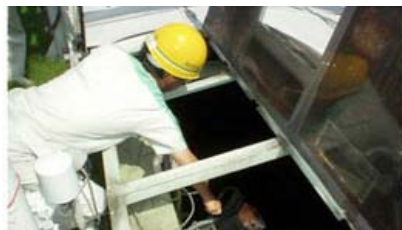
Shut down Emergency cutoff valve
