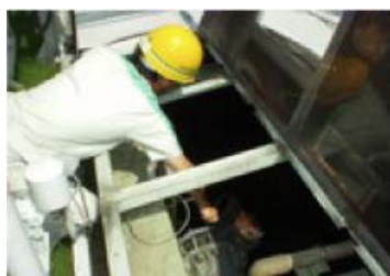
Shut down Emergency cutoff valve
