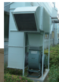
Exhaust vent with a noise reduction cover
