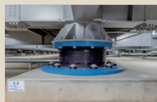
Sismic isolator
