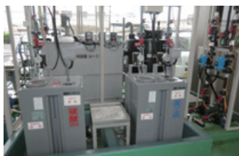
Neutralization segment of the industrial wastewater treatment facility
