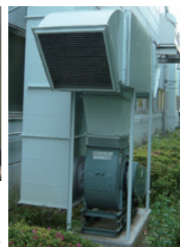
Exhaust vent with a noise reduction cover
