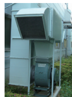
Exhaust vent with a noise reduction cover
