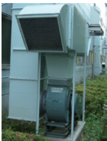
Exhaust vent with a noise reduction cover
