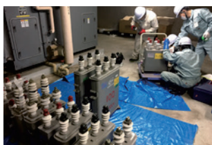
Transporting condensers containing PCB
