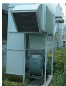
Exhaust vent with a noise reduction cover
