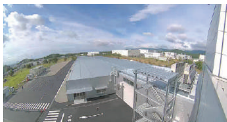
New building added to the second factory
