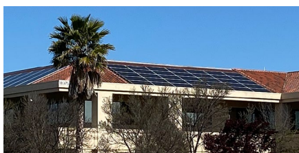
Solar power generation facilities
