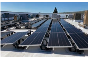
Solar power generation facility under construction at Morgan Hill
