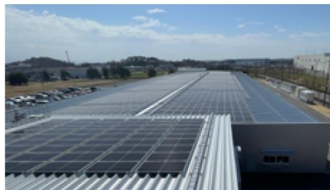
Solar power generation facility
