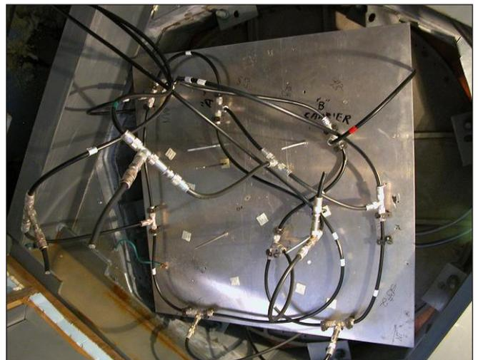
*Figure 7. Typical cabling installation in a VOR system is shown here. The system uses RG-214/U type coax and signal splitter/combiner components. Critical phase-matching requirements ensure the overall system operates correctly as a navigational aid for aircraft.*
