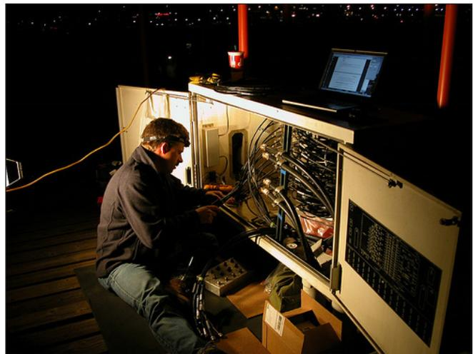
Figure 10. This system installation is configured with solid outer conductor cables. Maintenance activities are usually scheduled to avoid peak operational periods.
