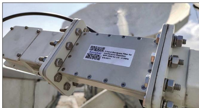
Figure 6. C-Band BPF Inserted into Feed Network
