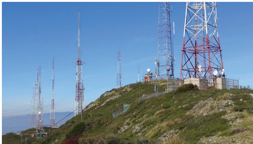
Figure 7. Multiple Co-Located Transmitter Towers often Result in Intermodulation between Signals
