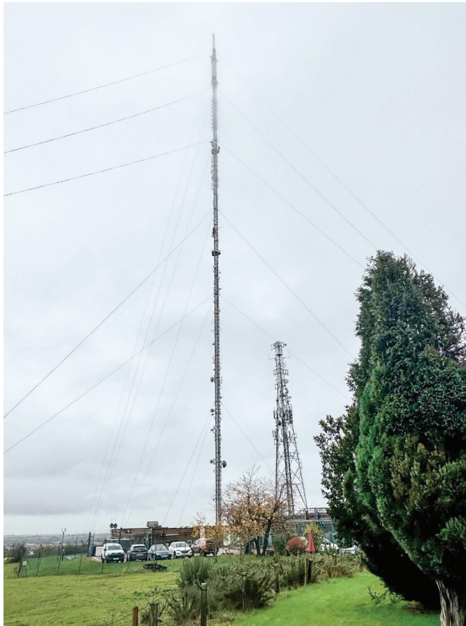
Figure 3. Transmitter Towers with High Power VHF Broadcast Radio and UHF Terrestrial Digital Television Transmitters Require Regular Testing to Monitor for Harmonic and Spurious Emissions
