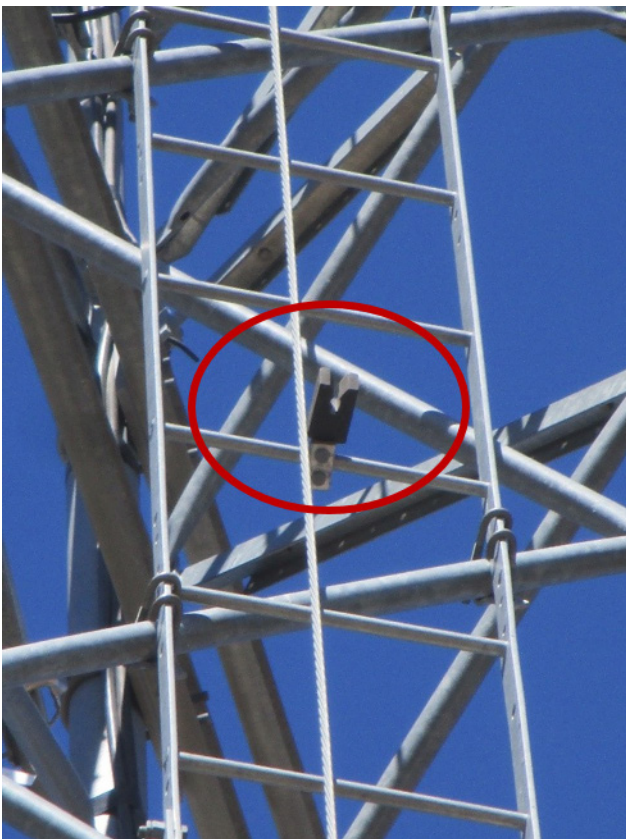
Figure 10. The safety climbing cable, shown having broken free from its isolating tower mount (left) and the loose metal chain (right) were both causes of PIM when being blown against the tower structure by wind.
