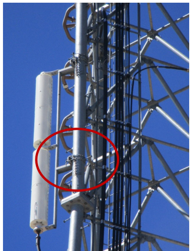
Figure 10. The safety climbing cable, shown having broken free from its isolating tower mount (left) and the loose metal chain (right) were both causes of PIM when being blown against the tower structure by wind.
