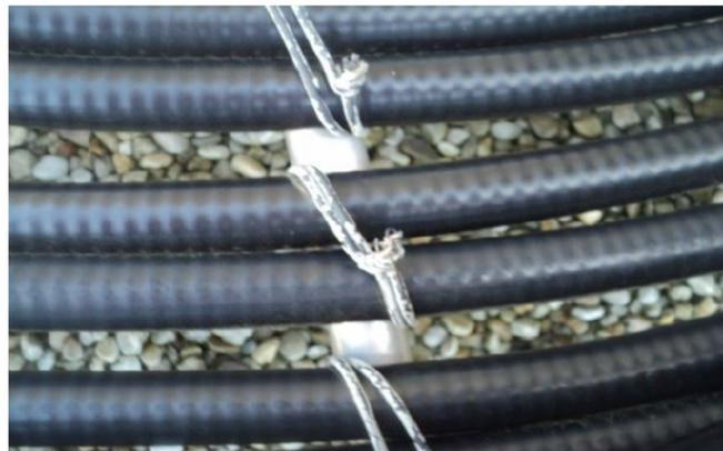
Figure 5. Improper Cable Camps
