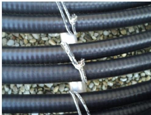
Figure 5. Improper Cable Clamps
