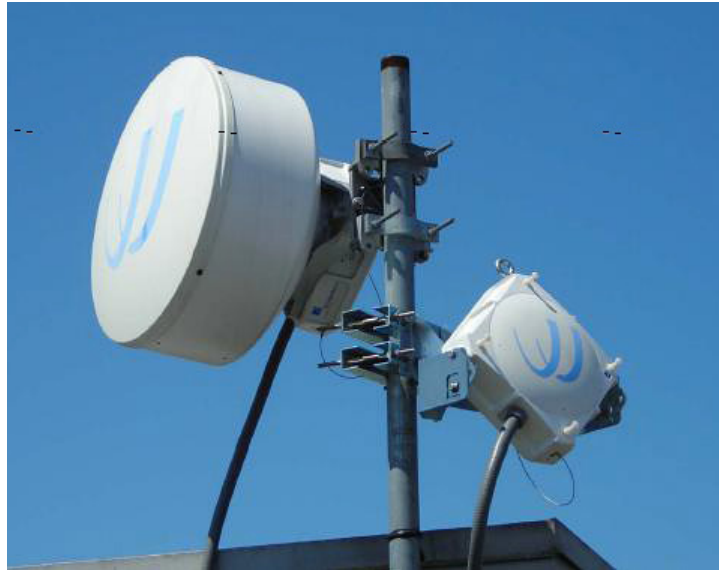
Figure 5. BridgeWave Communications 60 GHz unlicensed point to point radios links to MMW radios.
